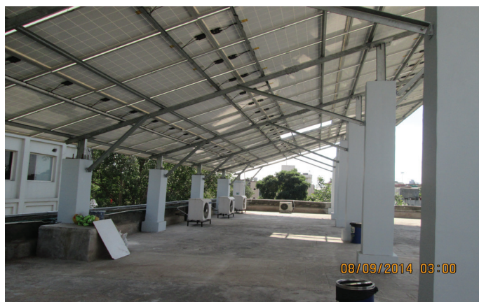
Figure 6.11: Canopy type mounting system
