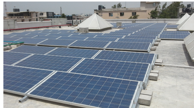
Figure 6.9: Ballasted roof mounting System
