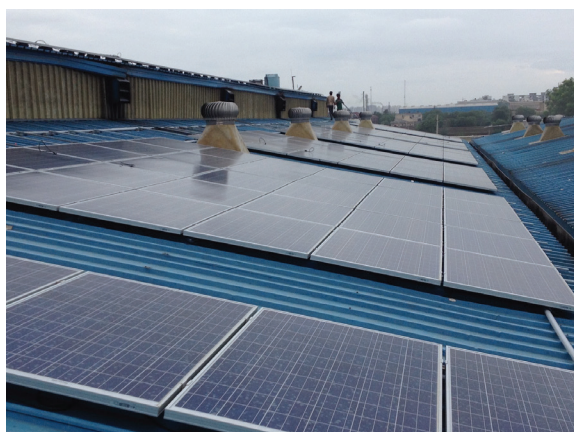
Figure 6.10: Mounting system for industrial sheds
