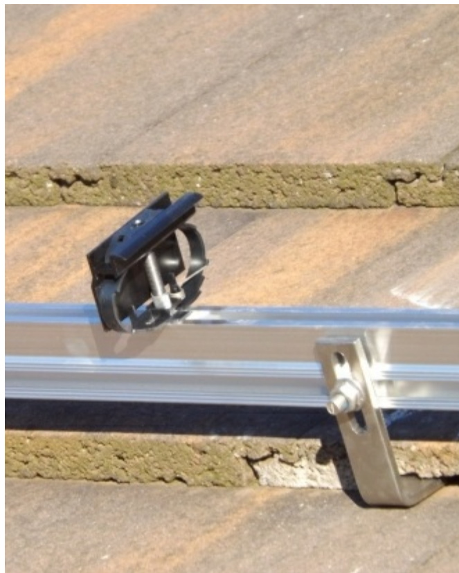
Above: Close up of a roof-mounted system, showing a roof hook, the mounting rail and a solar panel clamp.
