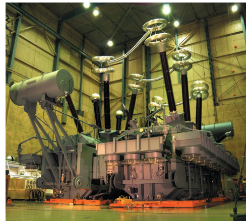
Set-up for three-phase induced test including partial discharge measurement.
